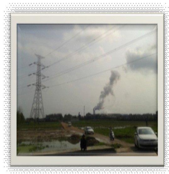
Fig 2(b) : Source of Pollution on Insulators from brick kilns
