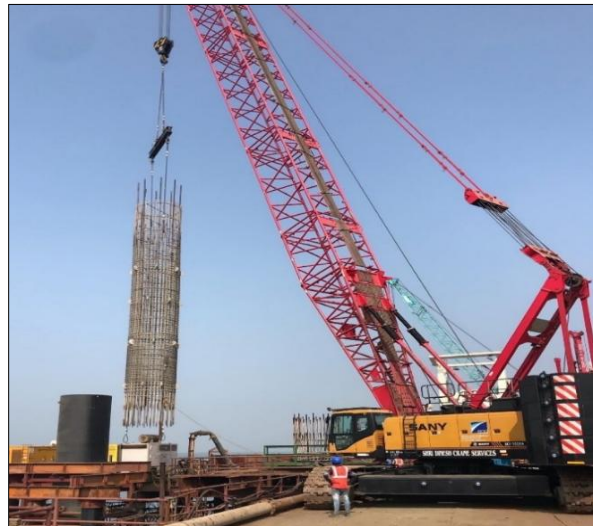
Figure 6: Rebar Cage Installation
