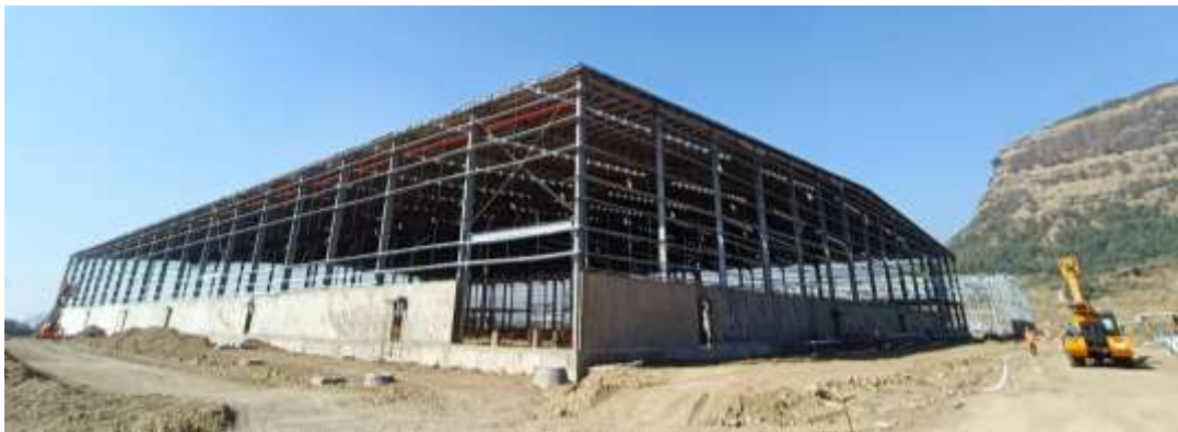
Figure 2: External View of the PEB Structure
